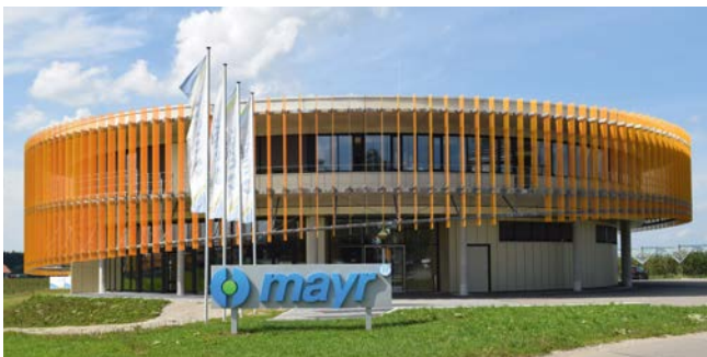
Communications Centre mayr.com – opened in 2018.
