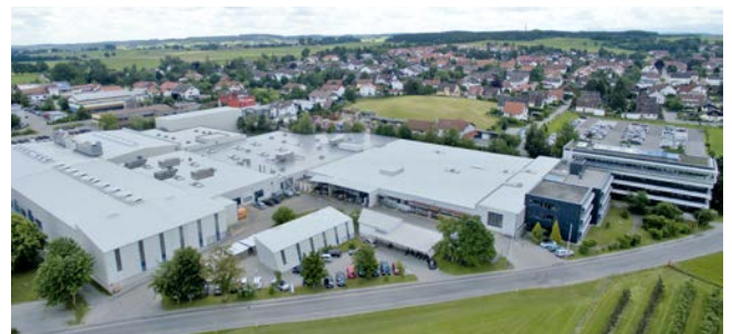
mayr ® -headquarters in Mauerstetten
